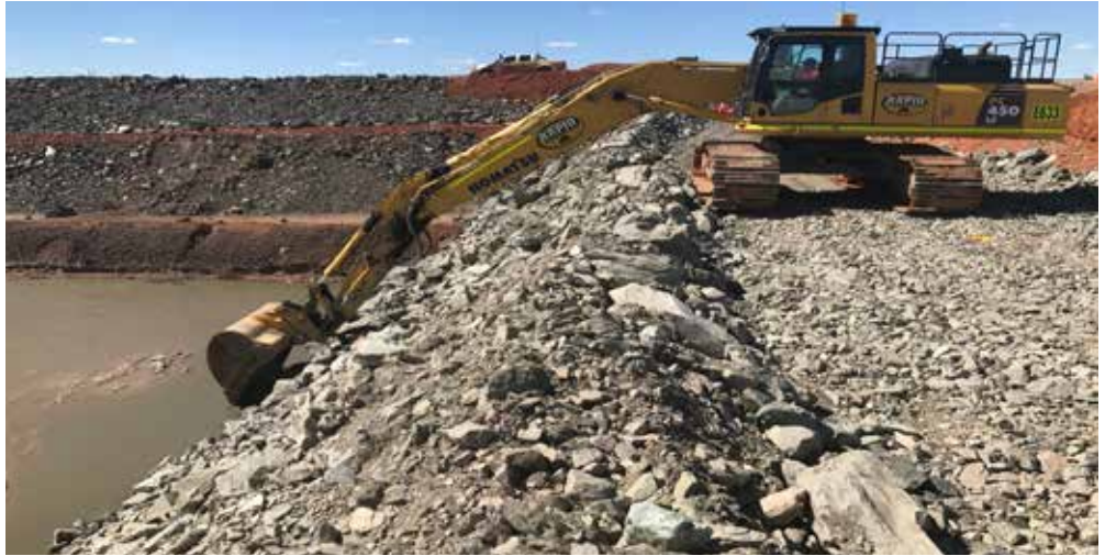
Rock Armouring on the Decant Access
