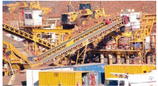
Modular crushing circuits on Burrup Peninsula
