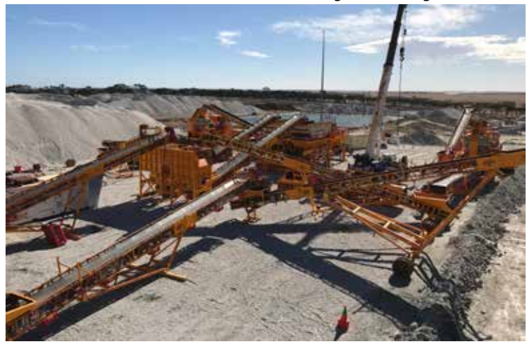
Below...The modular electric crushing circuit being installed
